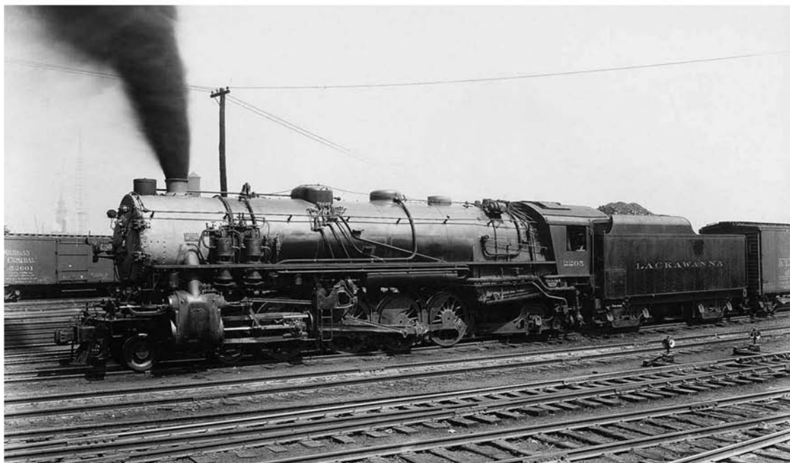
Delaware, Lackawanna & Western ordered two classes of three-cylinder 4-8-2s between 1925 and 1927. Five, numbered 1450 to 1454, were built for passenger service. No. 2205 was one of 35 built for freight service (Nos. 2201-2235). Thomas T. Taber collection Railroad Museum of Pennsylvania PHMC
