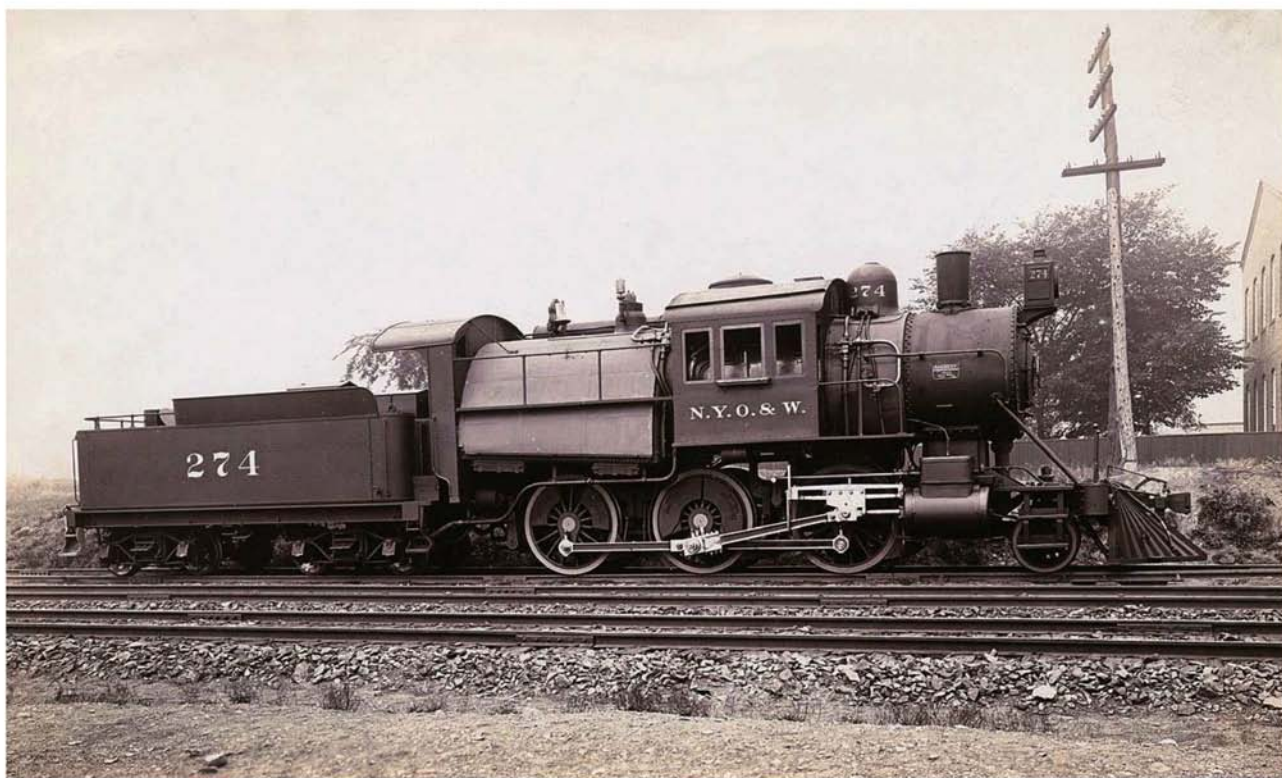
An Alco builder's card displays New York, Ontario & Western 2-6-0 camelback No. 274, built by the Cooke works in June 1908. On the O&W these were known as "Mother Hubbards." Anthracite burners used the broad, shallow Wootten firebox to obtain a satisfactory fire and draft. Thomas T. Taber collection, Railroad Museum of Pennsylvania PHMC
