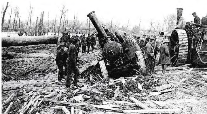
Left: Taken slightly later than the above photo, the Fowler engine on the right has moved forward, perhaps in readiness of hauling the other out of its predicament by using its wire rope. OLD GLORY ARCHIVE
