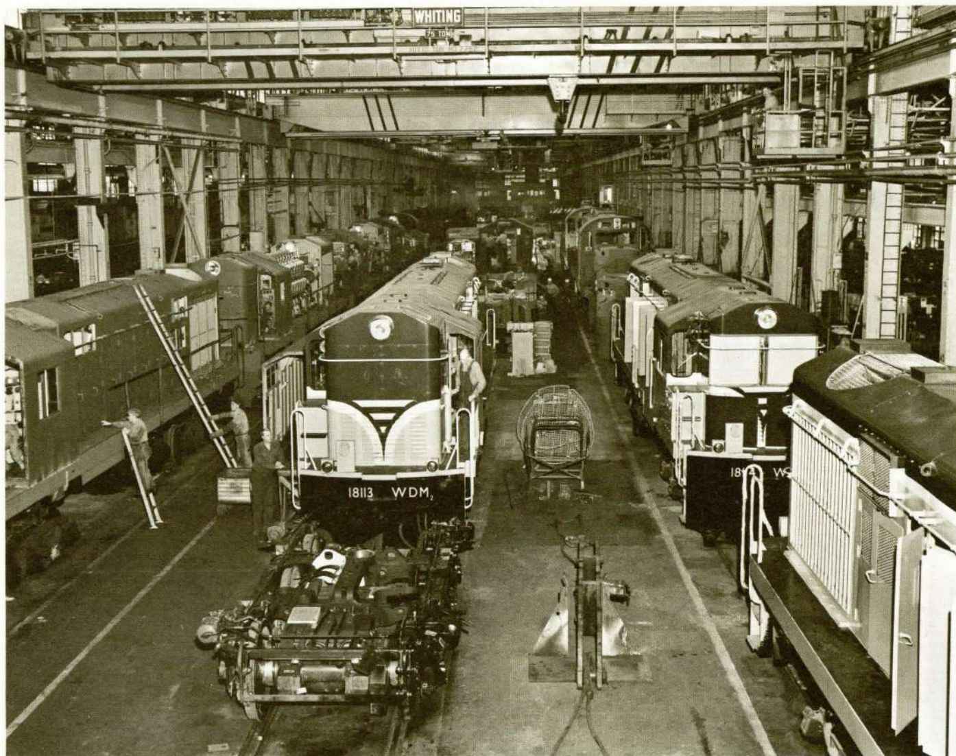
Modern facilities and new automation techniques are in evidence at ALCO—Schenectady, New York, the world's only straight-line, progressive-station locomotive assembly plant.
