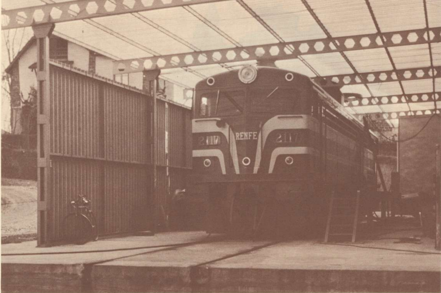
Finished locomotive on water box testing station for evaluation of power performance.
