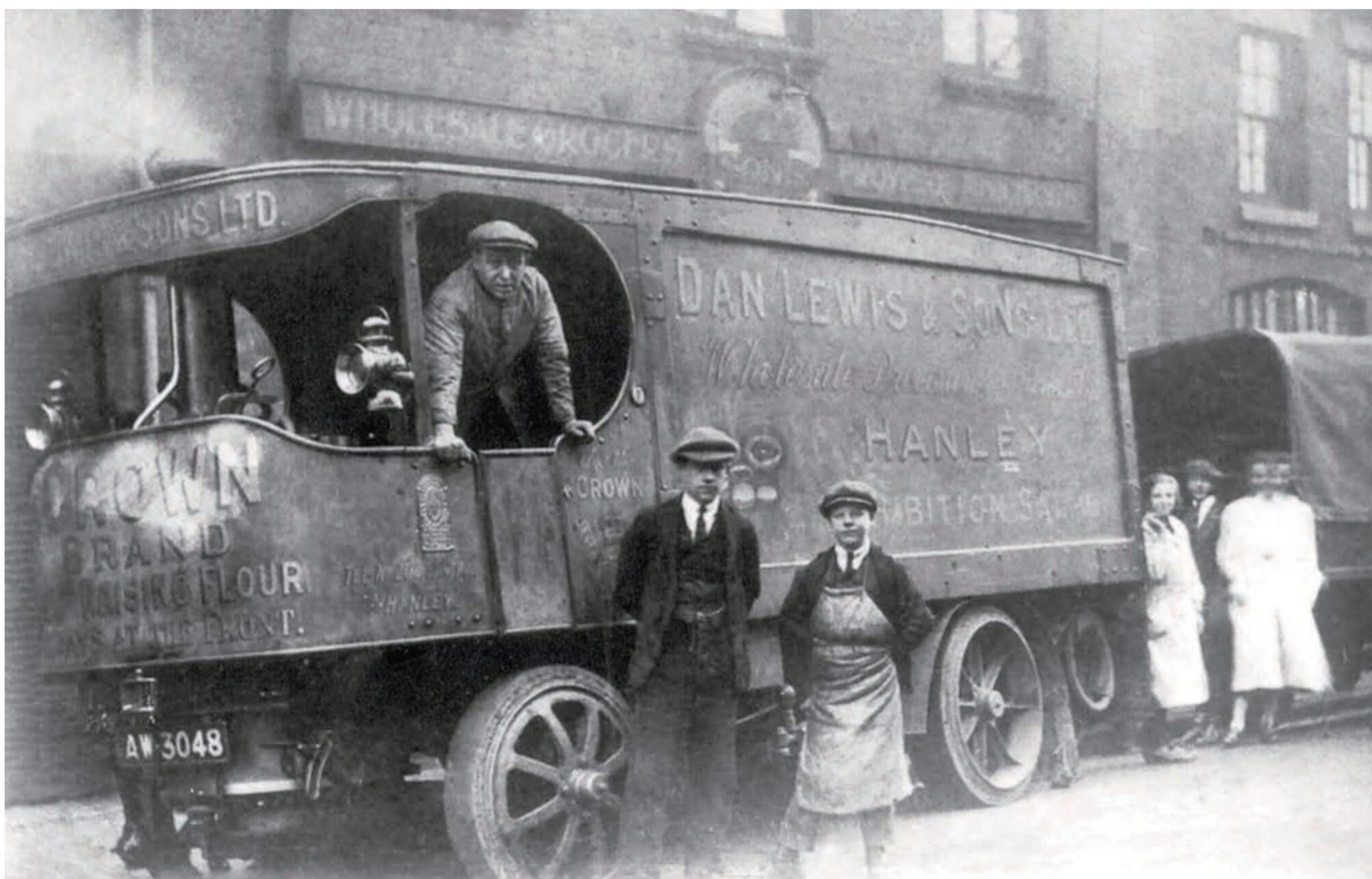
Fig. 3. Sentinel 3-ton Standard undertype waggon No. 1329 (AW 3048) was built c1916 and sold to Dan Lewis of Hanley, Stoke-on-Trent – a wholesaler that advertised Crown Brand self-raising flour on the front. It later sold to E.B Ward of Stockton Heath, Cheshire before passing to its last owner, Richard Allen of Widnes.
