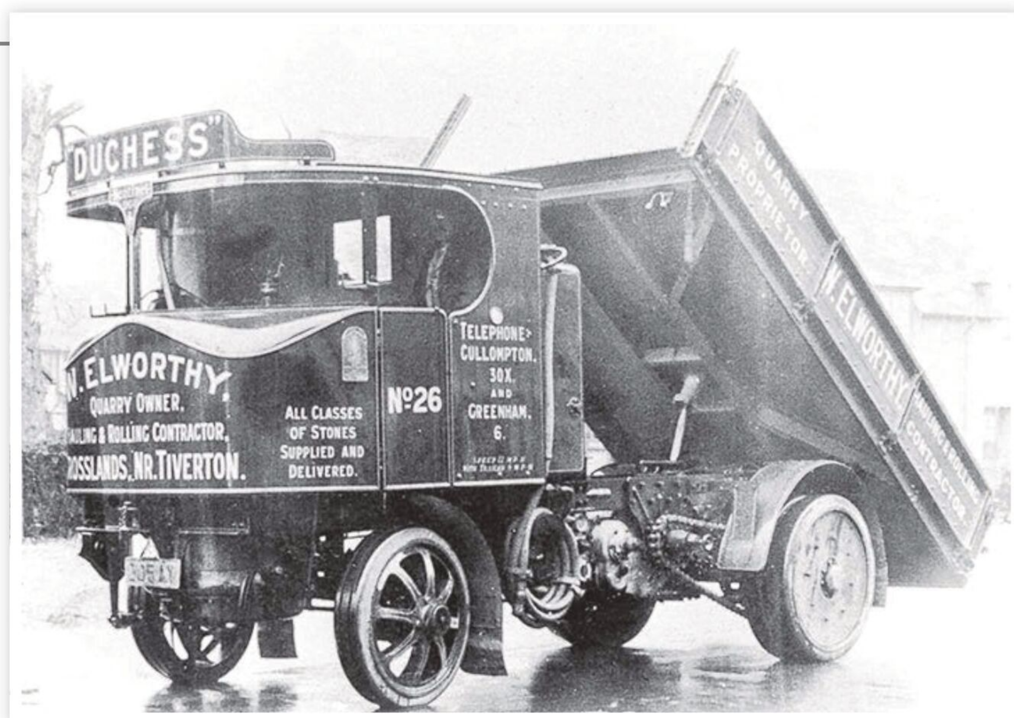
Fig. 8. Being demonstrated in the tipping position, Elworthy's quarry in Devon was the first recipient of DG4 tipper No. 8107.
