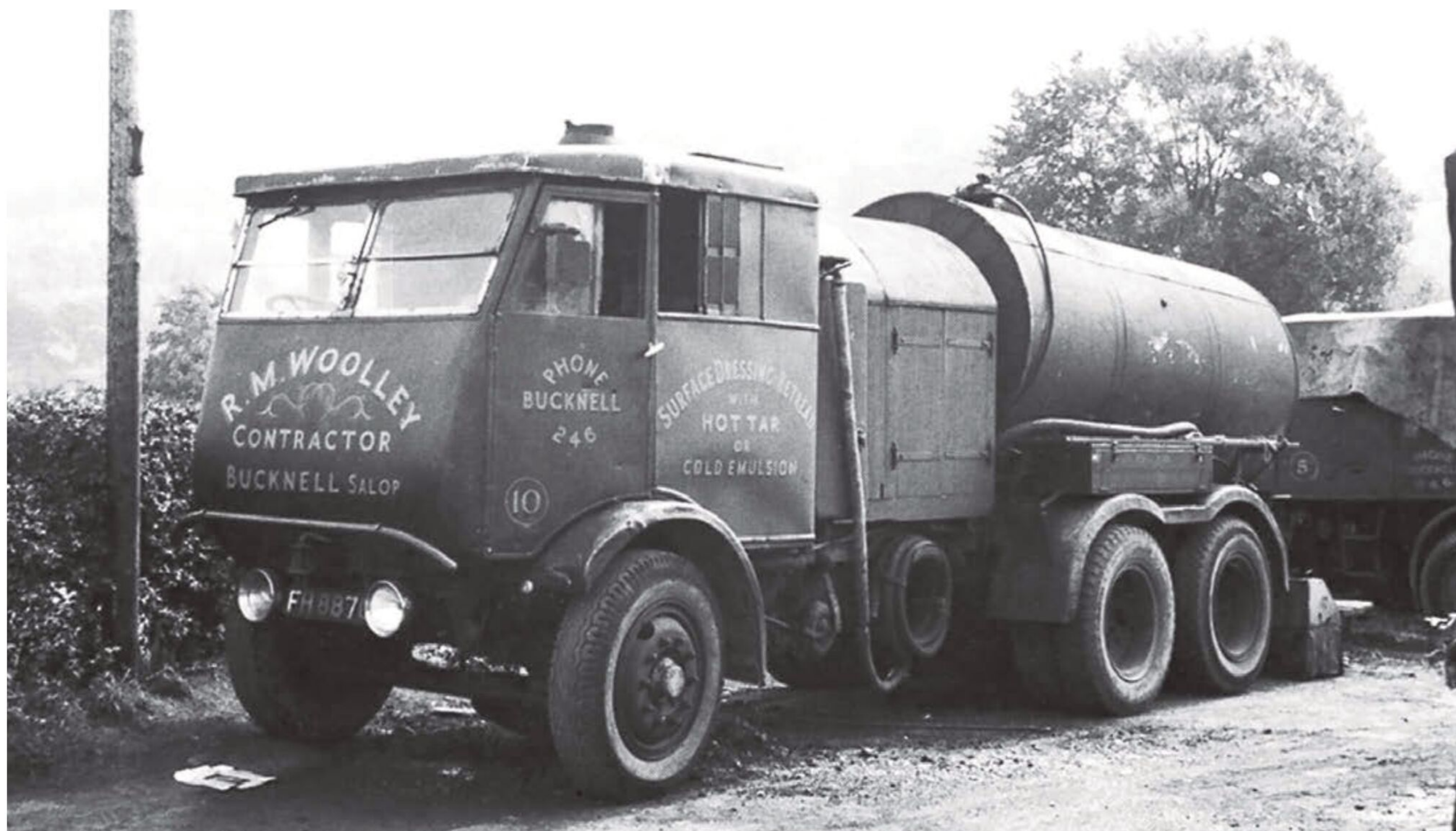
Fig. 9. S6 waggon No. 9084 of 1934 was fitted with tar spraying equipment.
