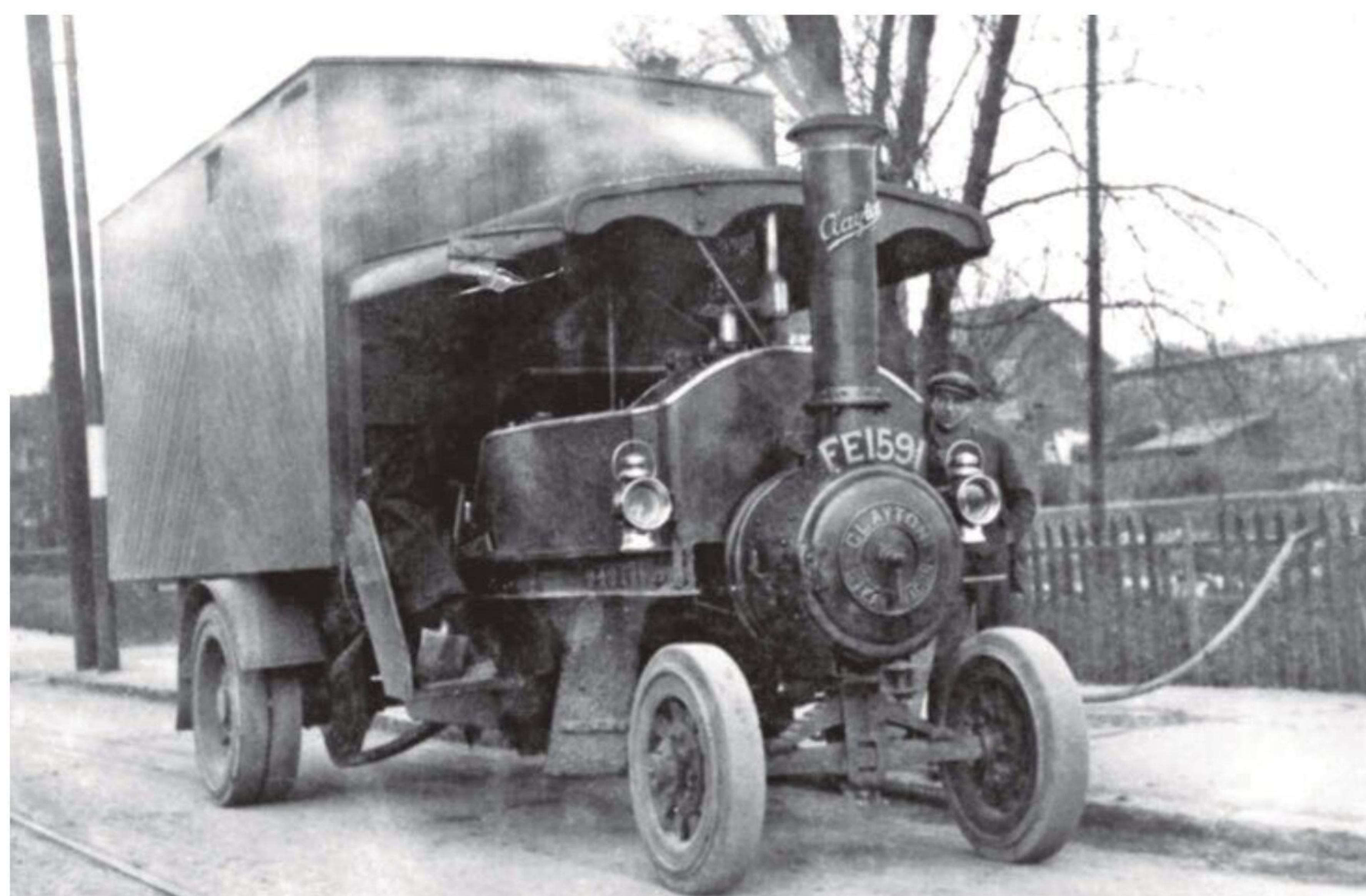
Fig. 6. Five-ton wagon No. 47136 takes water from a stream at Daybrook, Nottinghamshire c1917.
