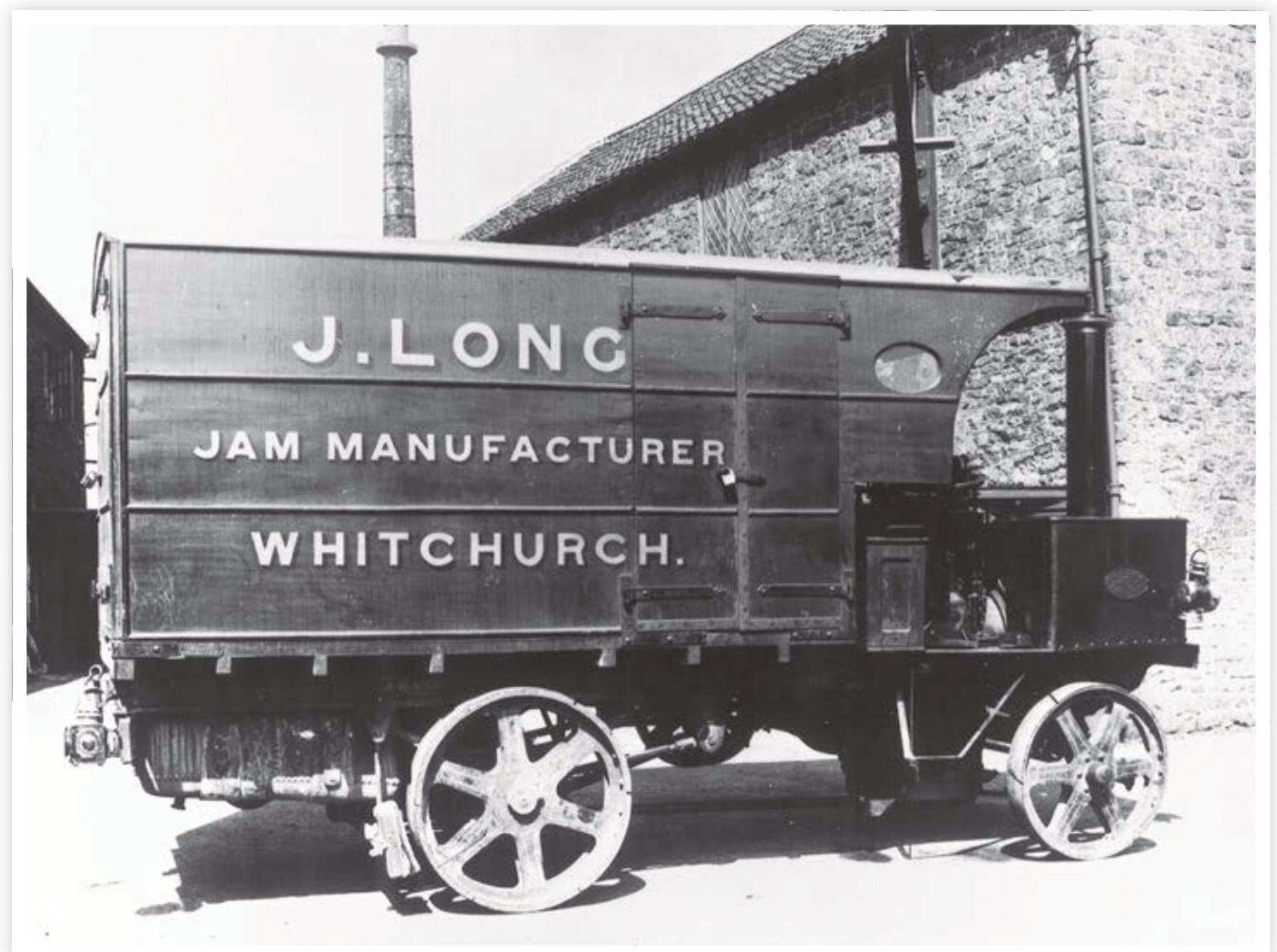
Hindley wagon fitted with an enclosed van body, built in 1907 and supplied new to J Long, jam manufacturers of Whitchurch, Hants. A 2-cylinder vertical compound engine was fitted on the rear of the vertical boiler.
