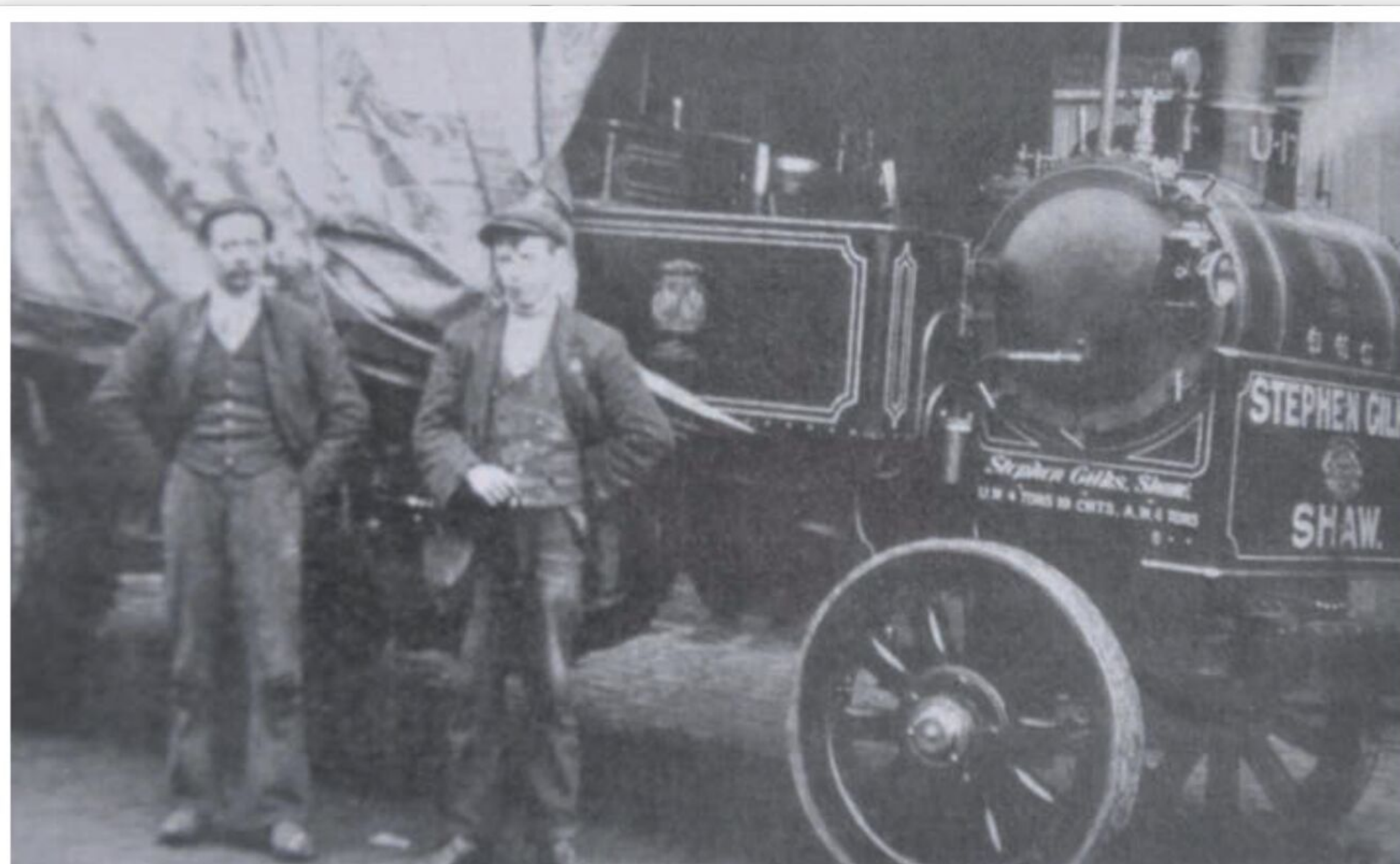
Fig. 3. Yorkshire wagon No. 142 with hand-operated tipping gear, the handle for which can be seen just to the rear of the cylinder.
